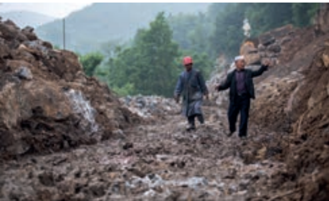
Top: An aerial photo shows a mountainous road zigzagging into the Kanzishan Village in Yunxi County, Hubei Province. Above: Wei Dengdian (R), Party secretary of Kanzishan Village, inspects the construction site of the road that leads to the village. Photos by Xiong Qi
