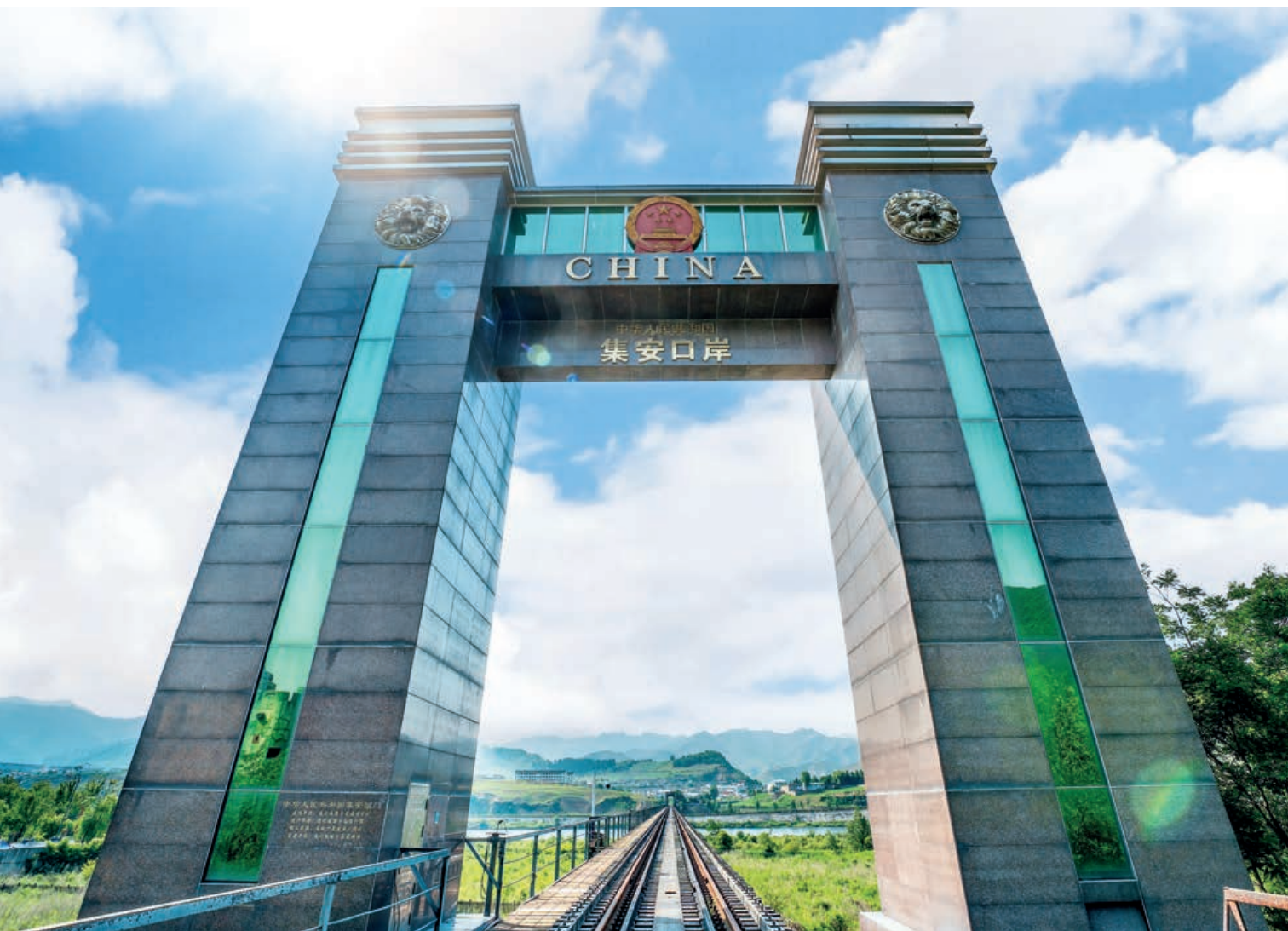
This photo taken on June 17, 2023 shows the Yalu River Border Railway Bridge in Ji'an city, northeast China's Jilin Province, which is at the border between China and the Democratic People's Republic of Korea. Zhou Wanpeng
