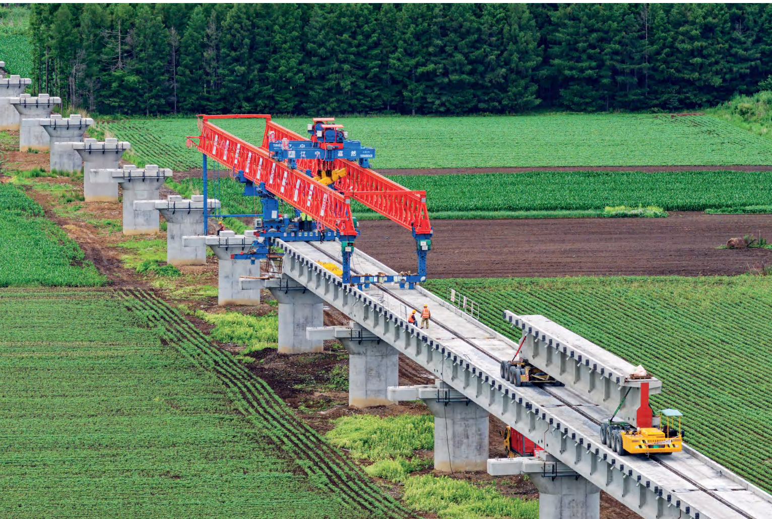
This aerial drone photo shows the construction site of the Tongjiang super major bridge, part of the upgrading project for the Jiamusi-Tongjiang Railway, in northeast China's Heilongjiang Province, June 25, 2026. The Tongjiang Port is a key gateway along the eastern corridor of the China-Europe freight train service. (Xinhua)
