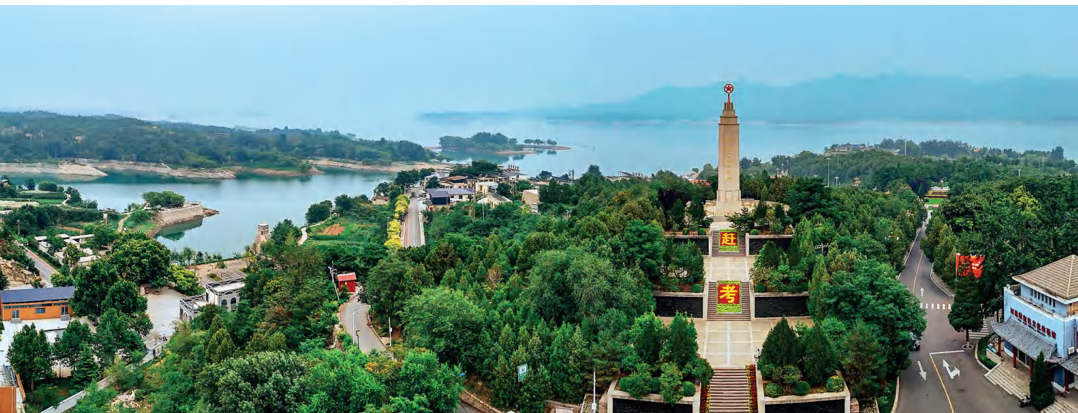
A panoramic view of the Xibaipo Memorial Hall. VCG
